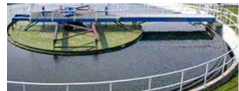
Effluent Treatment Plant with ZLD
